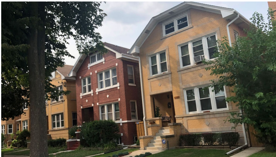
Much of the existing housing stock in Belmont Cragin is well-maintained but, due to age, might need structural improvements.
