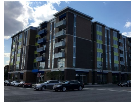
2900 N. Cicero 69 units 0.4 acres 5-Story Elevator Building 66,900 Square Feet 189 Dwellings/Acre Unit Mix: 1 Studio, 64 1-BR, 4 2-BR
