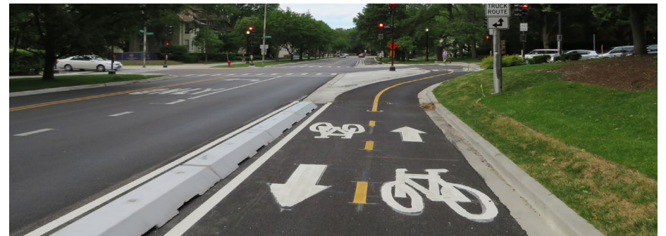
An example of a two-way, barrier-protected cycle track located in downtown Evanston.
