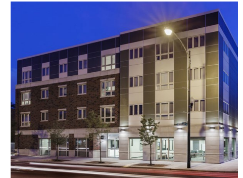
3060 N. Milwaukee Ave. 32 units 0.3 acres 4-Story Elevator Building 32,520 Square Feet 107 Dwellings/Acre Unit Mix: 25 1-BR, 7 2-BR
